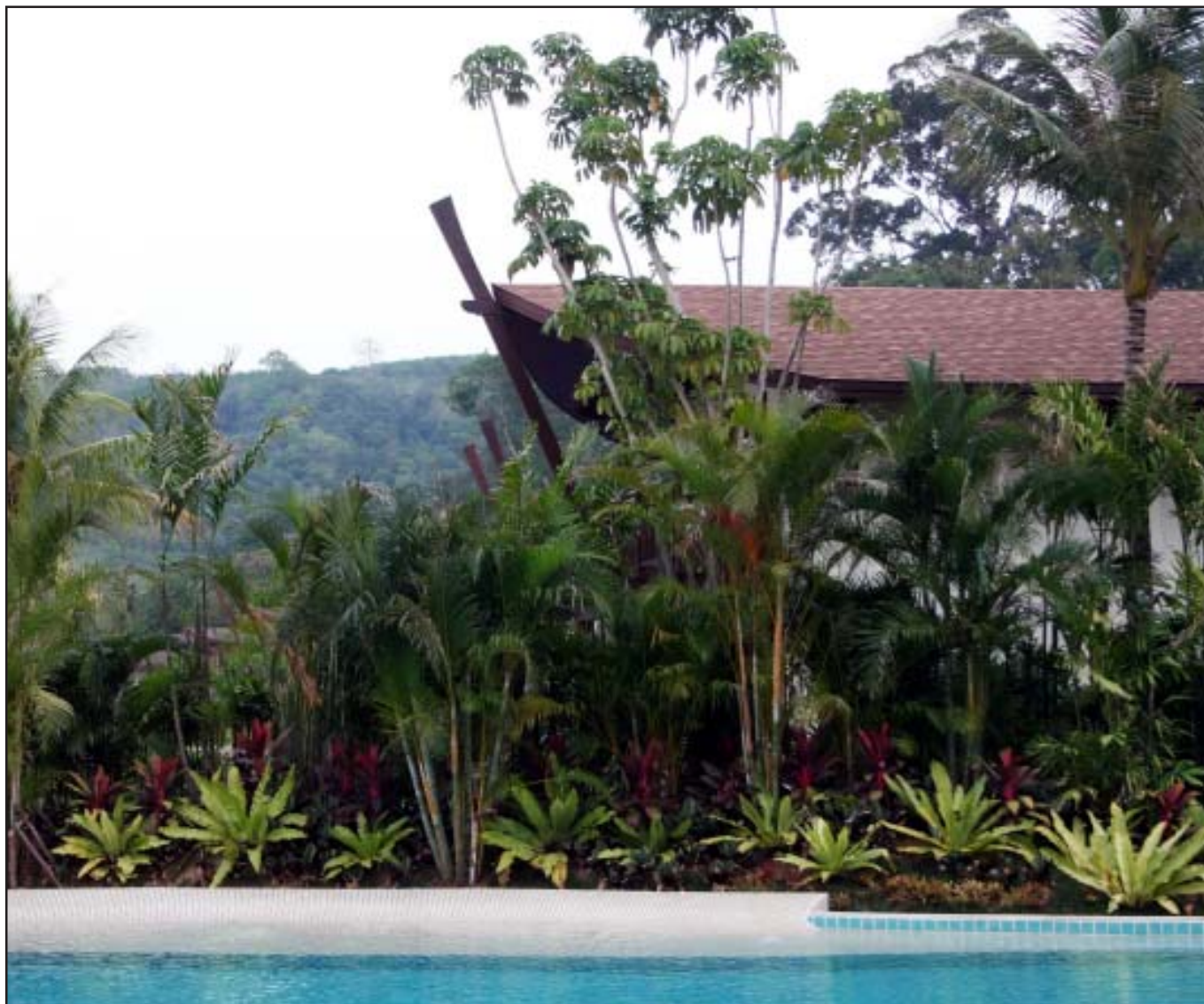
The roofs of The Village, apart from lending a Thai taste to the homes, are also practical
